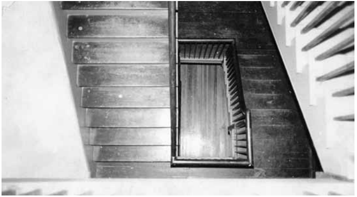
Figure #2 Stairwell from Attic Floor
