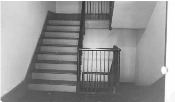
Figure #5 Second Floor Hall
