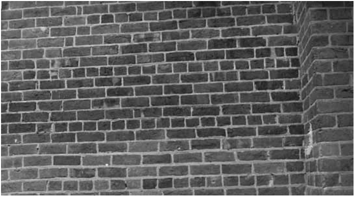
Figure #1 Exterior Brick Work Pattern
